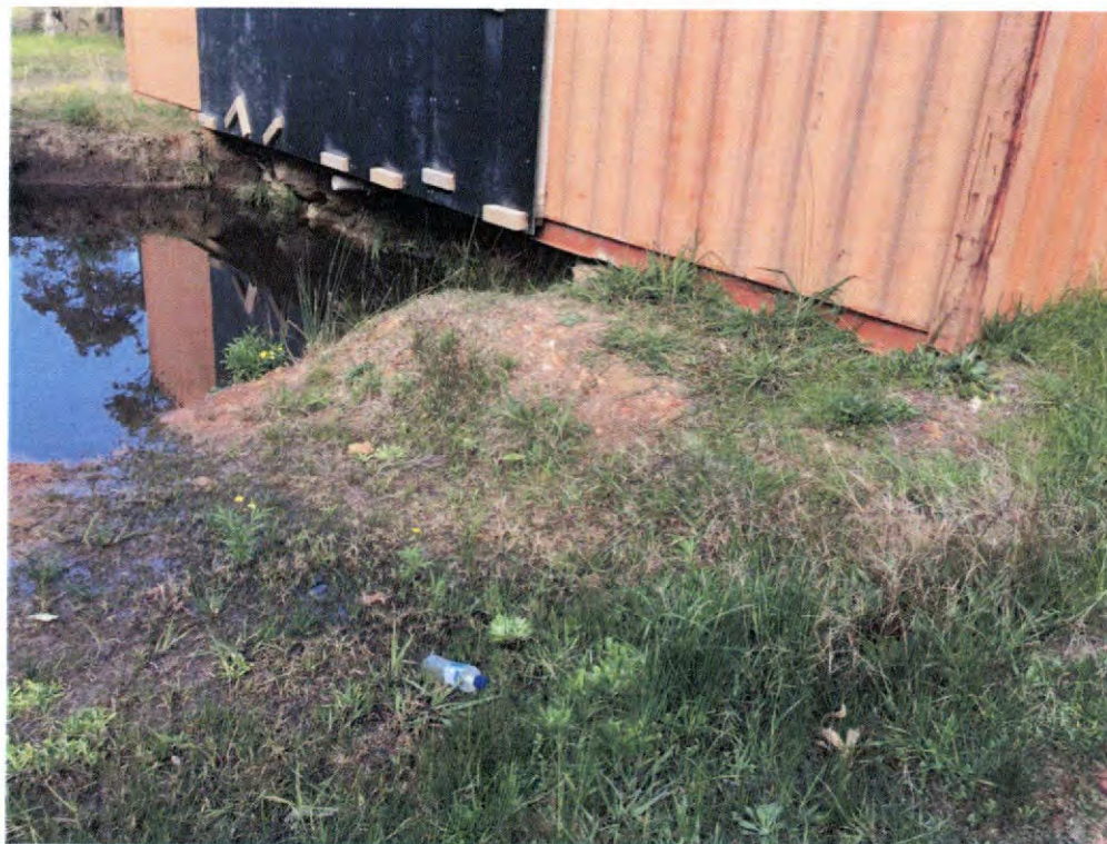
PHOTOGRAPH 12 The use of fill before or during the construction of the obstacle/ assault course.
