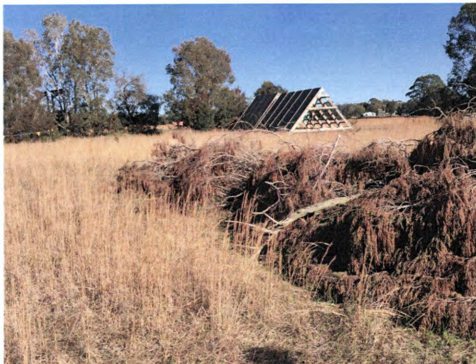
PHOTOGRAPH 3 General site topography and outlay- northern corner of the site, looking south west.
